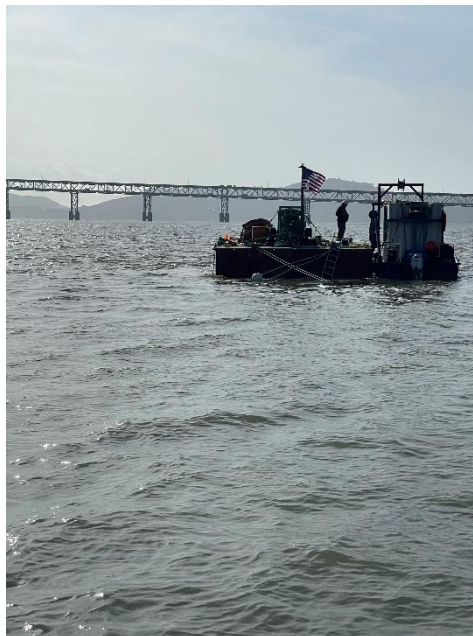
Photo 4: Contractor's Barge Platform at Diffuser No. 115
