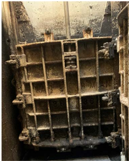
Originally installed cast iron sluice gate
