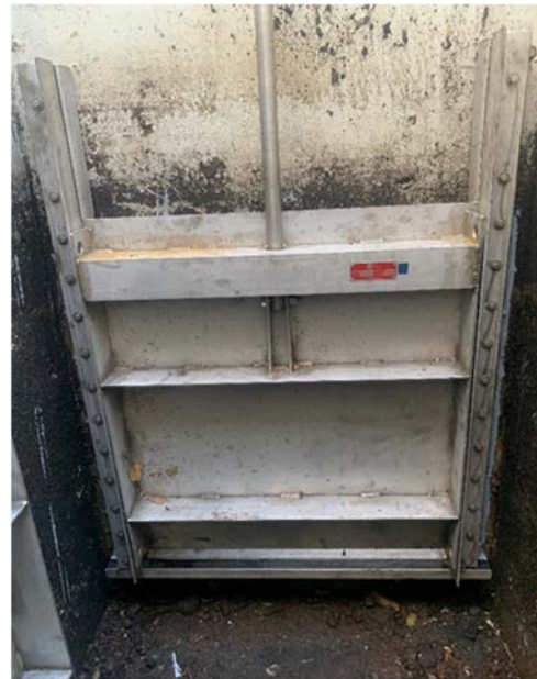
Recently installed stainless steel sluice gate
