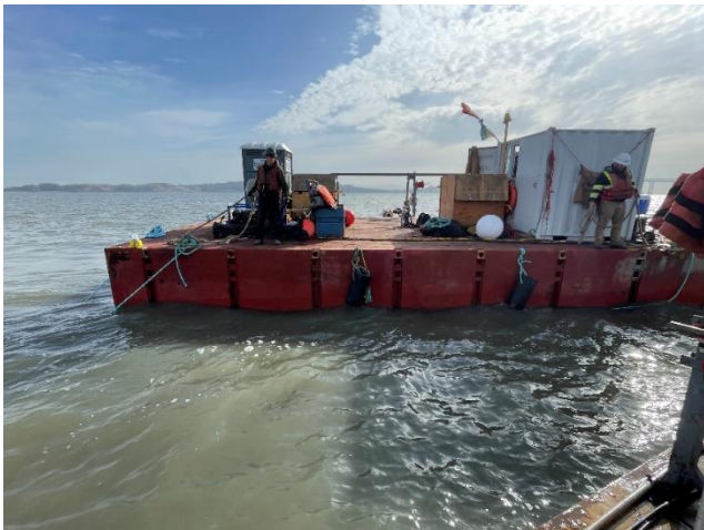
Photo 3: Contractor's Barge Platform at Nearshore Access Manhole
