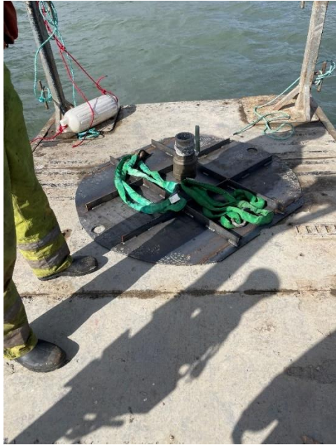
Photo 6: Temporary Cover for CMSA Nearshore Access Manhole
