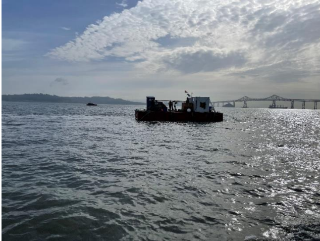
Photo 1: CMSA Outfall Diffusers Section Location in San Francisco Bay
