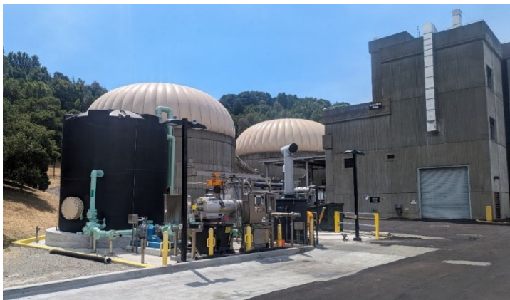
Completed Liquid Organic Waste Receiving Facility
