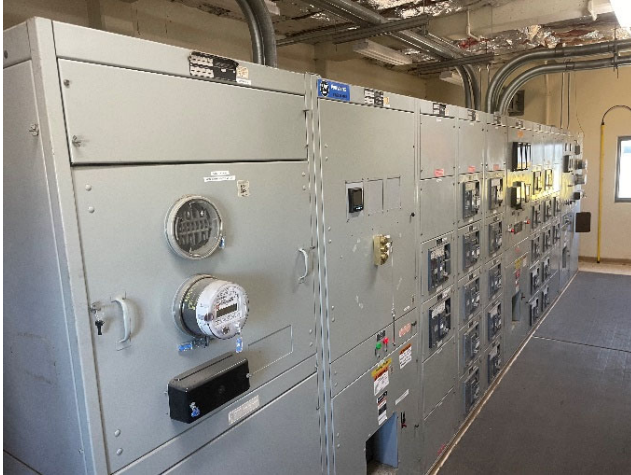
Main switchgear.
