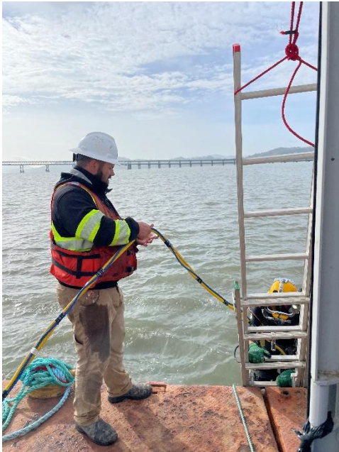
Photo 7: Diver Exiting the Nearshore Access Manhole
