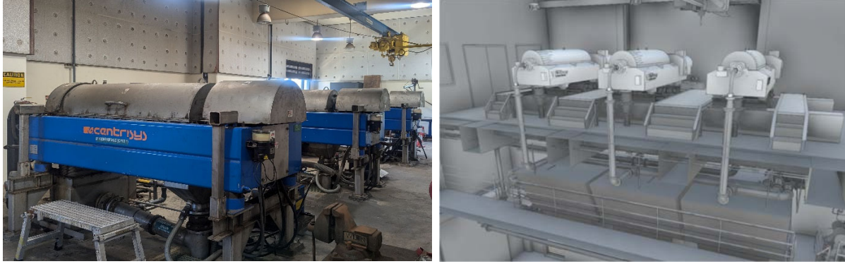
Existing Centrifuges (left) and 3D Model of the centrifuge room with the new centrifuges (right)
