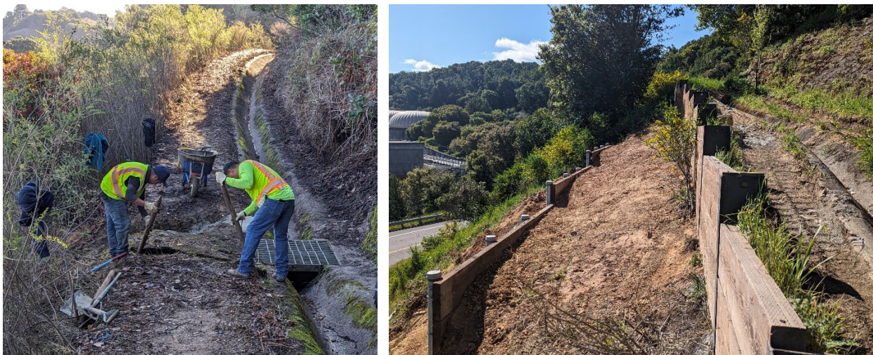
V-ditch Maintenance (left) and New Retaining Wall (right)
