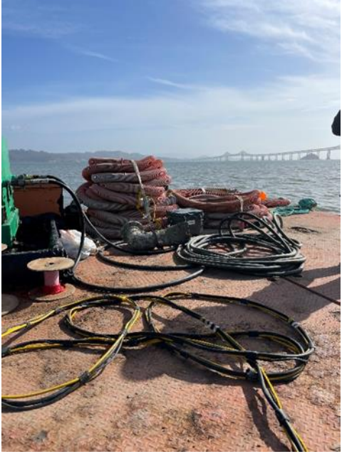
Photo 8: Barge Platform with Removed Duckbill Diffuser and Hoses
